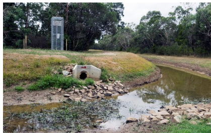
Above: The catch drain and the diversion structure. Below: The pipe flowing into the Devilbend Creek bed below the catch drain
