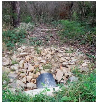
Above: The catch drain and the diversion structure. Below: The pipe flowing into the Devilbend Creek bed below the catch drain
