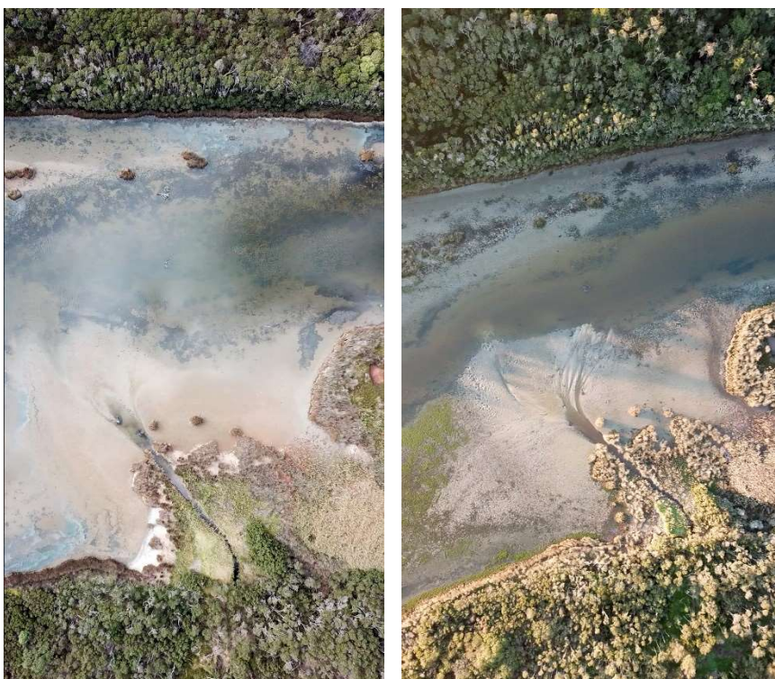
Drone images of the plume from the Henley Avenue stormwater drain discharge point: Left, March 2018; Right, June 2019 Images by George Murley
