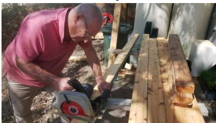
Above: Hard at work on the fence frames.
