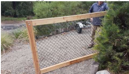
Below: Ready for installation Photos Suzanne Ryan
