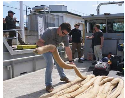
Sandbag 'snakes' loaded onto a barge, to be used in the Corner Inlet project. Source: ABC Gippsland: Peter Somerville www.abc.net.au/news/2019-11-01/fighting-urchin-induced-seagrass-devastation/11658504
