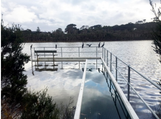
Above: Cormorants perched on the flooded rotunda jetty on the morning of 4 th May. Below: Seepage from behind the berm, 31 st May; Bottom of page: Sandy beach for miles! – looking north from North Beach carpark
