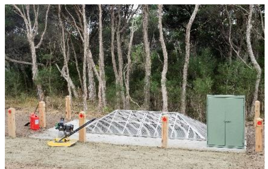
Installation of the Henley Ave baffle pit:
