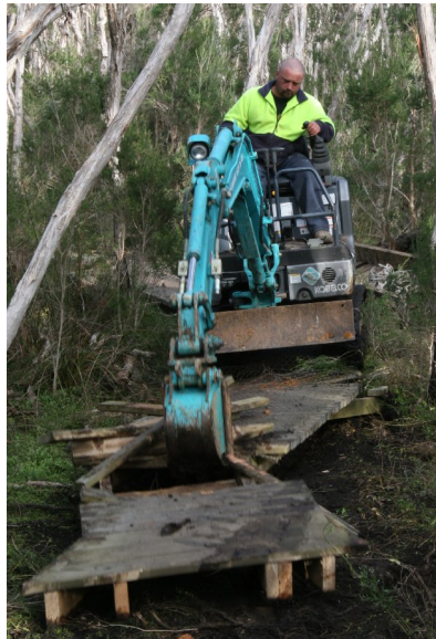
At work removing the old board walk!
