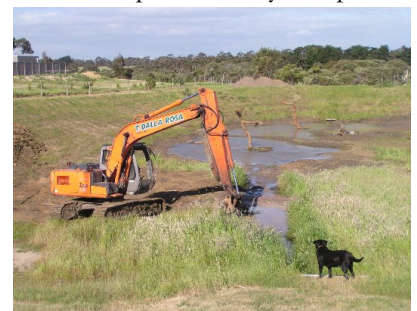
An excavator with an audience! – creating the new Century Drive Wetland
